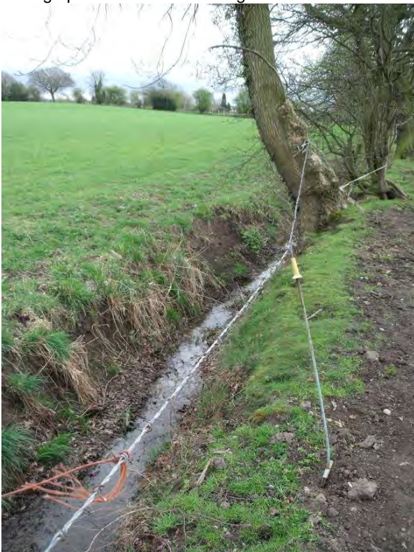
Photograph 17: View south along drain.
