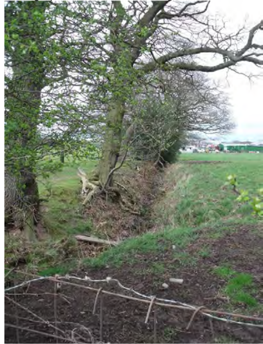
Photograph 20: View north along drain from outfall pipes.
