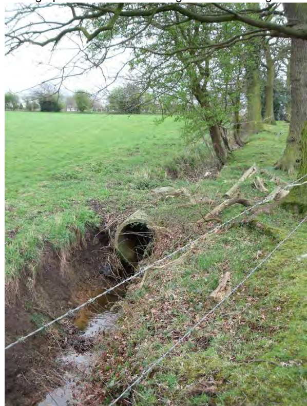
Photograph 18: view south along drain at existing culvert.
